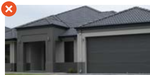
Garage should not be level or in front of the main house
